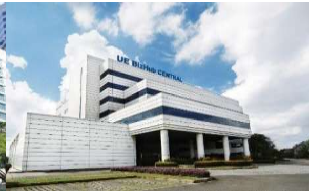
UE BizHub CENTRAL (as PPE) Industrial & Office GFA: 36,076 sqm (388,315 sqf)
