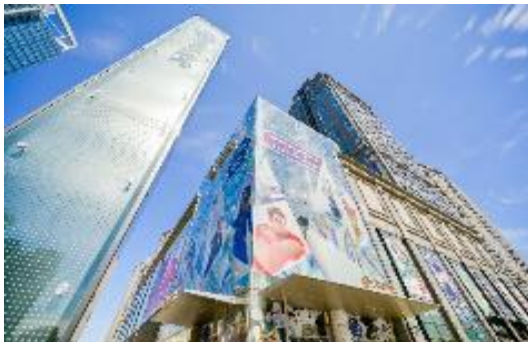
Yanlord Riverside Plaza, Tianjin 仁恒海河广场，天津 ▪ Office, Retail Mall & Commercial Street ▪ Total GFA: 159,807 sqm
