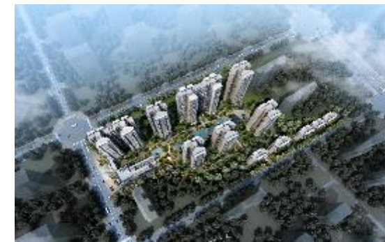
Yanlord Begonia Park (Phase 3), Haikou 仁恒海棠公园三期, 海口
