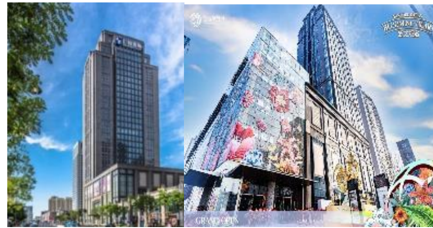
Yanlord Riverside Plaza, Tianjin 仁恒海河广场, 天津 Office, Retail Mall & Commercial Street Total GFA: 159,807 sqm Reopening of shopping mall on 30 September 2021
