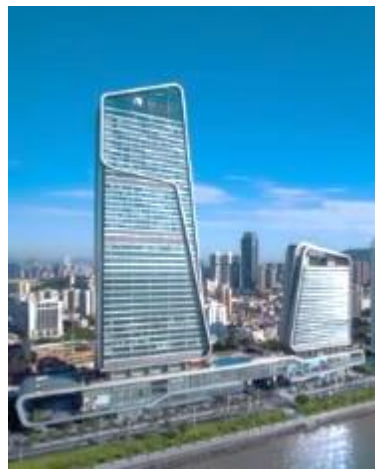
Yanlord Marina Centre, Zhuhai 仁恒滨海中心, 珠海 Office & Retail Total GFA: 42,974 sqm
